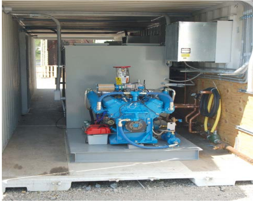
Figure 3. Tecogen Prime Mover with Inverter
