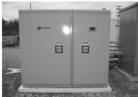
Figure 5. S & C Static Switch (from their Purewave product).
