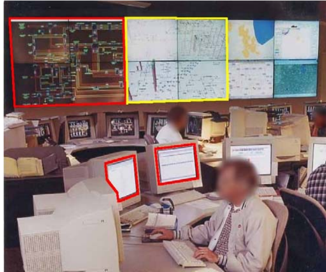
Figure 1. A power system control room with traditional tabular and static wall-mounted displays (outlined in red) and a new, three-dimensional graphical one-line display (outlined in yellow).
