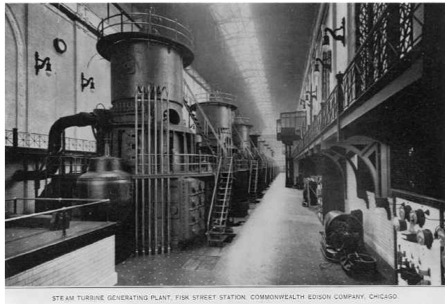
Figure 2-11 - Fisk Street Station, Commonwealth Edison Co., Chicago [37]
