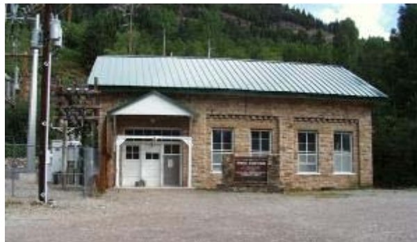
Figure 2-6 - Ames Power Station, near Telluride, CO (today)
