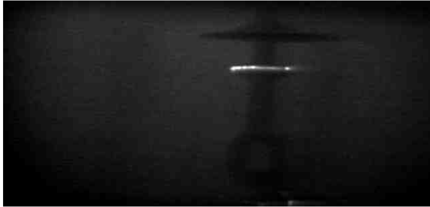
Figure 3: Corona at 50 KV of discharge magnitude 30 pC
