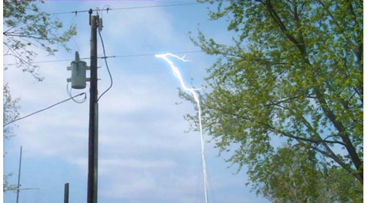
Arc between electric line and the ground.
