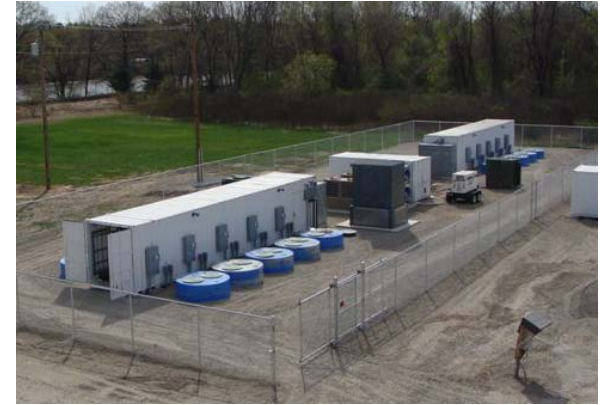
2-MW flywheel storage in ISO-NE (Source: Beacon Power)
