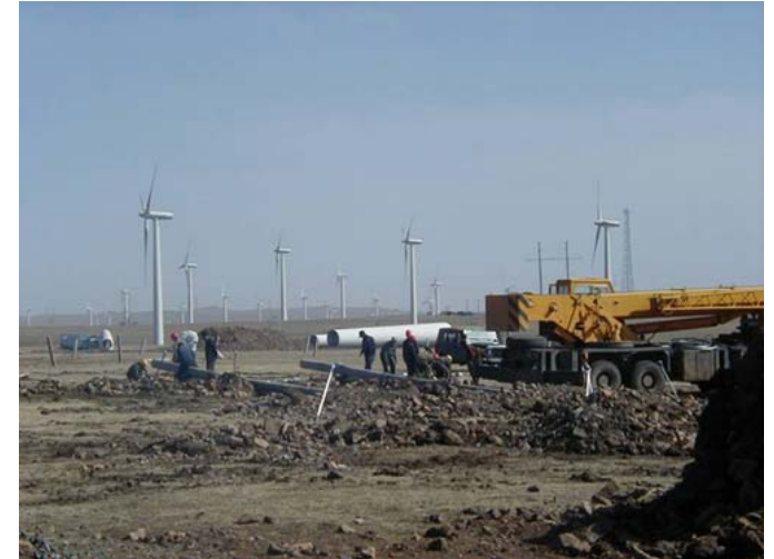
Wind farm under-construction
